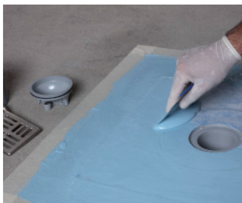
Impregnating Drain Vertical fabric with Mapelastic AquaDefense Zero
