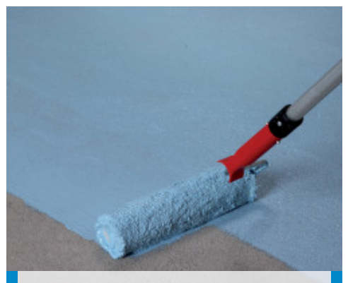
Application of the first coat of Mapelastic AquaDefense Zero on a screed
