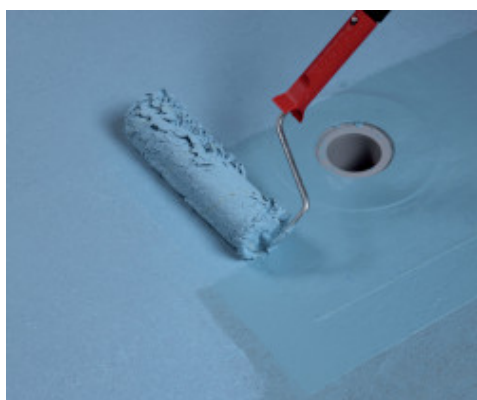
Application by roller of the second coat of Mapelastic AquaDefense Zero
