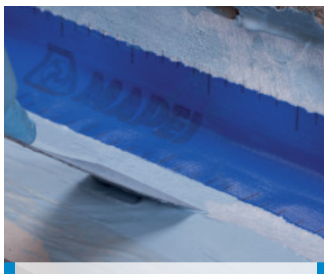
Application of Mapeband on a wall-floor fillet joint with Mapelastic AquaDefense Zero
